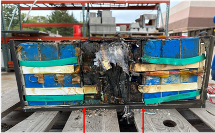
GORE Battery Insulation placement
