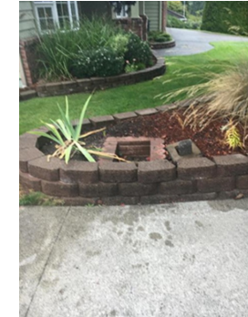
Landscaping Burying Meter
